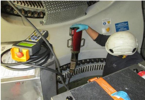
Figure 9: alkitronic® EF 300plus on a rotor blade
