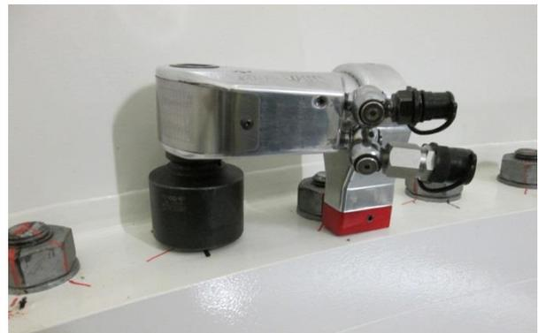
Figure 4: alkitronic® Hydraulic torque wrench AS-3 on tower flange bolts M36- high tension
