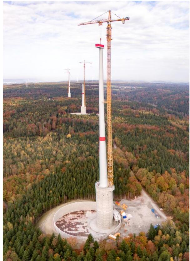
Figure 3: One of the wind turbines under construction. Foto: © Max Bögl Wind AG, photographer: Holger Hessenthaler.
