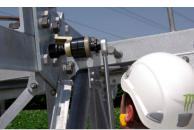
**alkitronic® M-HG** operating on electricity pylons. Accurate tightening via torque wrench.
